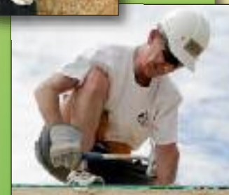
Ken Pinkham nails down second-story flooring
