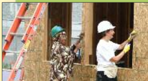
Future homeowner Farthiya Jilo and Karen Pinkham frame out windows
